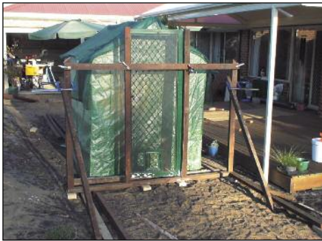
Photo 1: Starting by, getting the front of the frame in position and braced.
