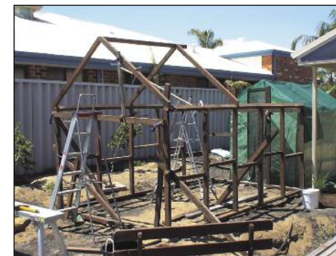
Photo 4: Constructing the roof using "A" frames .
