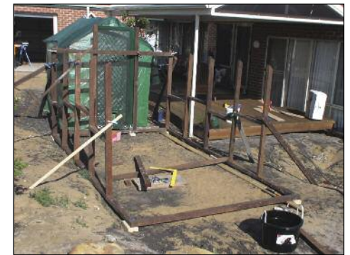
Photo 3: Putting up the side wall.
